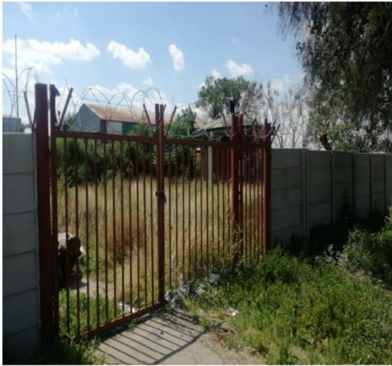
Power weg pump station
