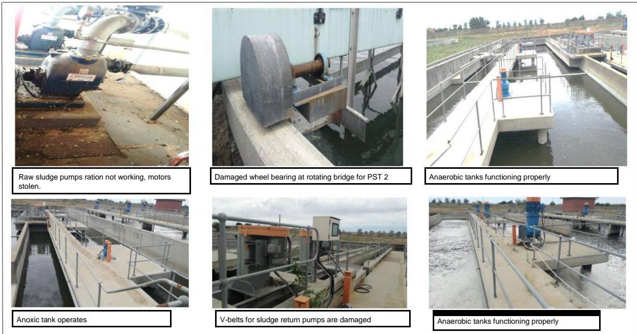
Thabong WWTW (continued)
