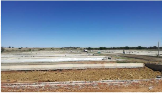
22 drying beds, currently under refurbishment
