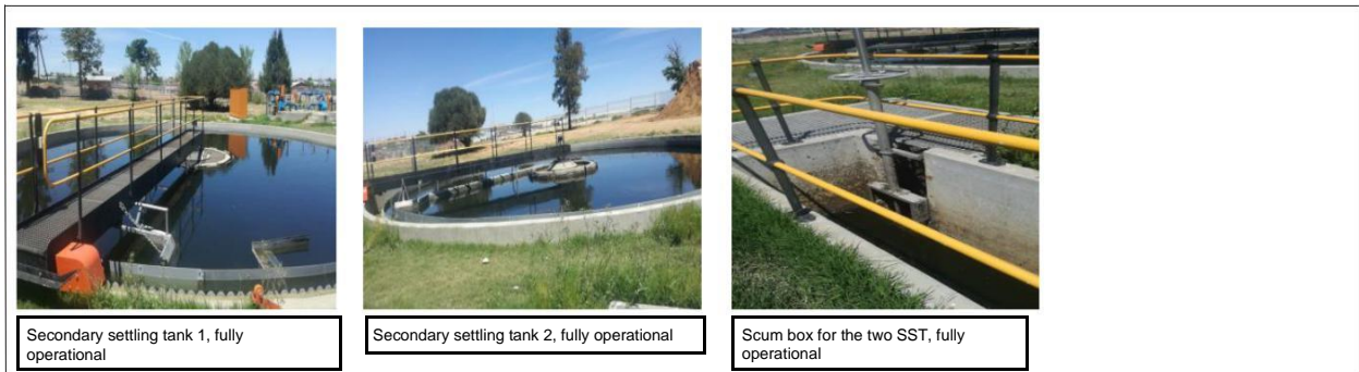
Nyakallong WWTW (continued)
