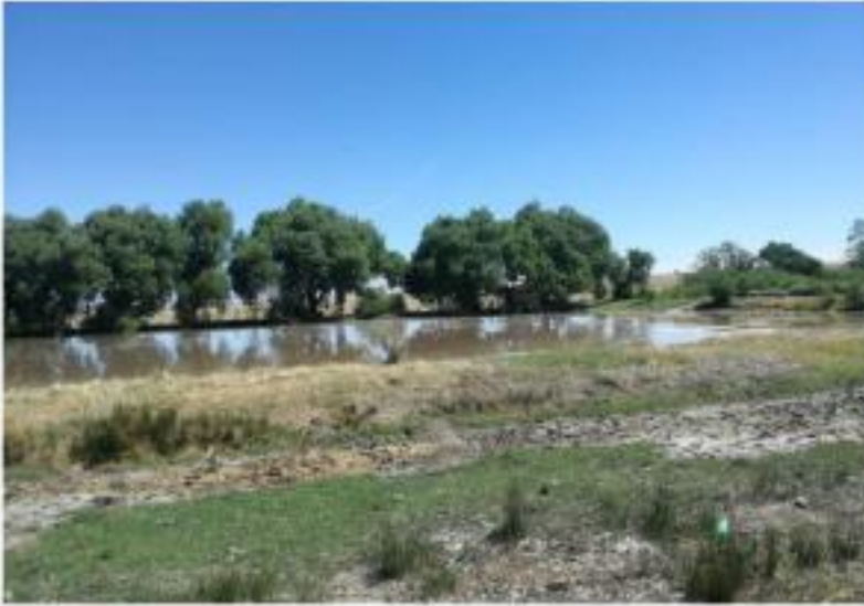
Oxidation pond, self purification plant, only has 4 oxidation ponds. Pond contains blood from the abattoirs
