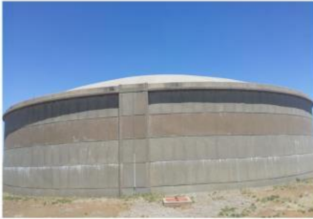
Ventersburg reservoir, no faults were found
