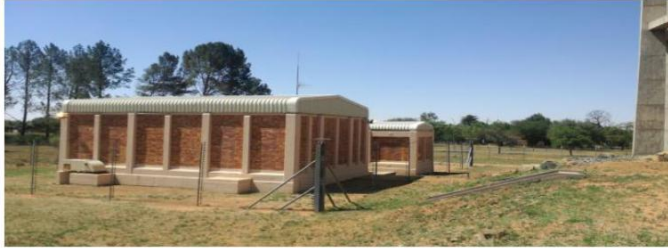
Pump station at Allanridge, pump working
