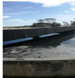
Theronia WWT (continued) : All the above pictures are the primary settling tanks (pst's). There are nine of them in total. There are all not working and old.
