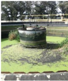
Theronia WWT (continued) : All the above pictures are the primary settling tanks (pst's). There are nine of them in total. There are all not working and old.
