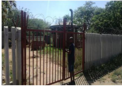
Verkeer Pump Station
