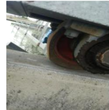
Damaged wheel on secondary sedimentation, SST 2 bridge
