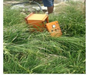
Panel box fully operational
