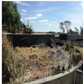
Theronia WWT (continued) : All the above pictures are the primary settling tanks (pst's). There are nine of them in total. There are all not working and old.
