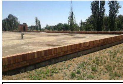
Allanridge reservoir, no issues
