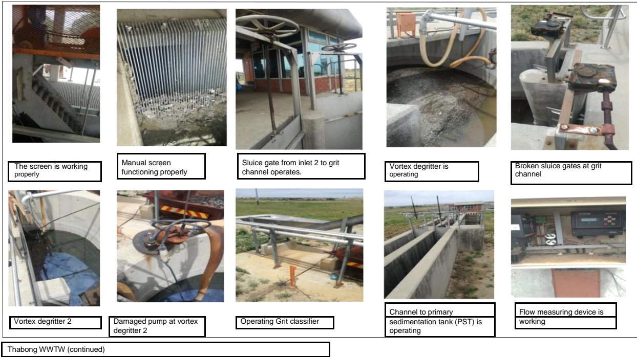
Thabong WWTW (continued)
