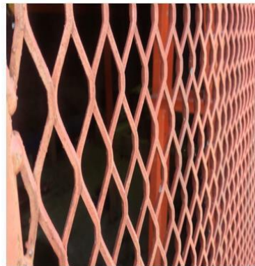
No key, no pumps inside. Contractor to do refurbishment on this Pump station
