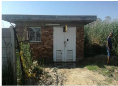
Western pump station
