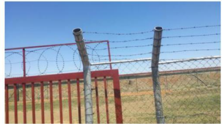
Dirksburg 1 and 2 are divided by a brick wall
