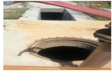
Channel to sumps
