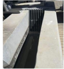
Manual screen, fully operational
