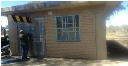
Building entrance is in good condition
