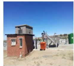
Overall view of mamahabane pump station
