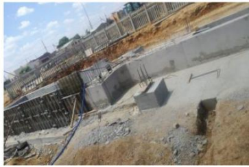
Under construction, plant being expanded increase the capacity
