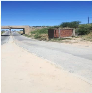
Subway Pump station
