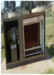
Vandalised transformer.
