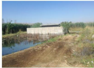
Lots of cable theft has occurred here
