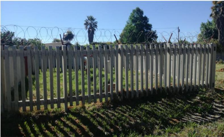
Hertzog pump station
