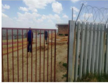
Thabong T8 pump station gate
