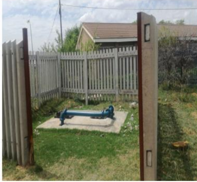
Eldorie Pump station, no gate
