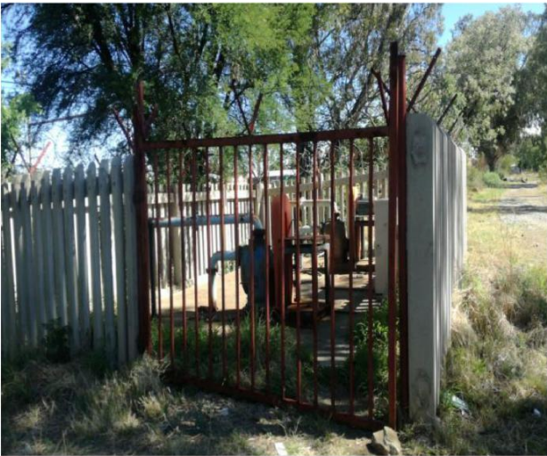
External view of the pump station
