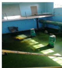
Electrical connection stripped due to cable theft, no electricity at all.
