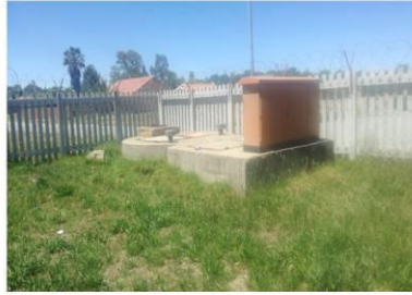
Temporary pumps inside the manholes working
