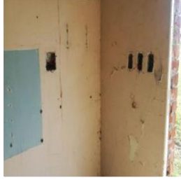
Electrical connection stripped due to cable theft, no electricity at all.
