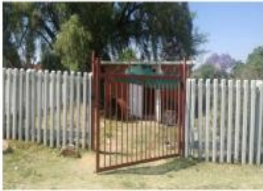
Rheederpark pump station
